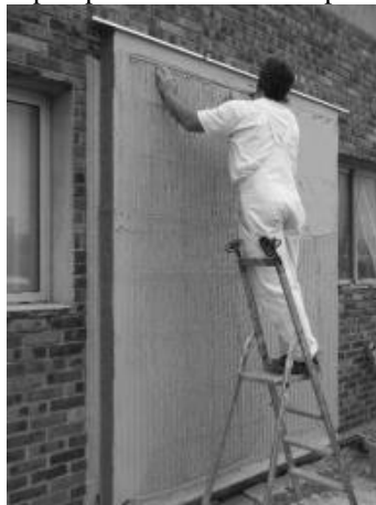
Fig. 3 Capillary tubes within a render finish [2]
